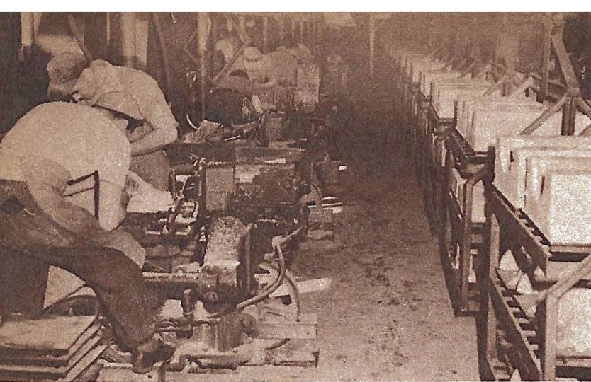
Left: A production line in the foundry of the Wright Aeronautical Corporation, Fairlawn, N. J., where cylinder heads for Wright Cyclone engines are cast on a mass production basis for National Defense. The airplane companies need skilled foundry workers.
