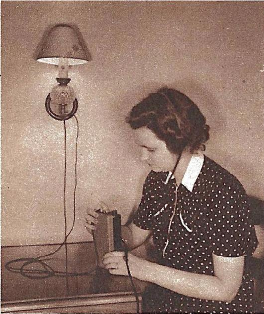
A piece of flexible wire clipped to the electric fixture makes an effective aerial for Pocket Pete.
