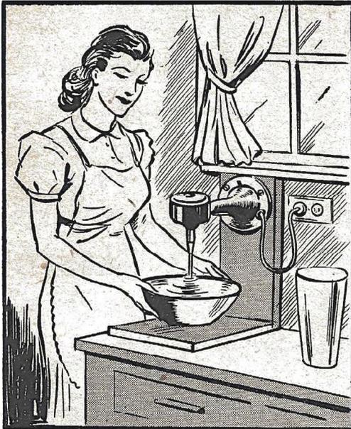
The head of the mixer tilts back to permit placing of bowls, shakers, etc., underneath. Drawing at right shows two different types of mixing arms.
