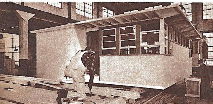
Here's the house assembly line. The cottage shown is almost completed, and the workman in the foreground is working on the floor platform of another.
