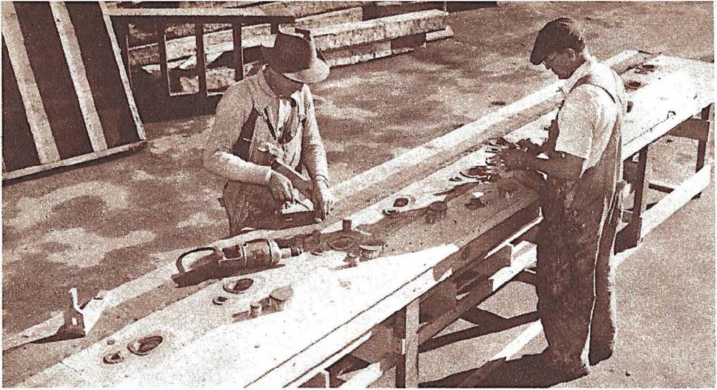
Walking through sand, the ghost left feminine footprints. Here those prints are being made on a 30-foot board, with wood and lead plugs fitting into the cut out "feet." The board was covered with sand, the plugs were dropped from below, and presto—the ghost walked!
